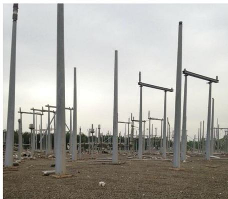
Entergy Arkansas' Mayflower substation, one of the three major substations serving the Little Rock area, suffered heavy damage in the April 27, 2014 tornado. The 500-kV high-voltage yard lost all of its switches and breakers. (Source: National Weather Service (left), Entergy (right))
