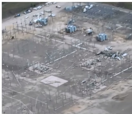
Entergy Arkansas' Mayflower substation, one of the three major substations serving the Little Rock area, suffered heavy damage in the April 27, 2014 tornado. The 500-kV high-voltage yard lost all of its switches and breakers. (Source: National Weather Service (left), Entergy (right))
