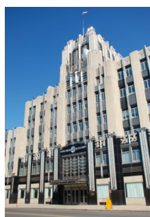
Niagara Mohawk building in Syracuse, N.Y.
